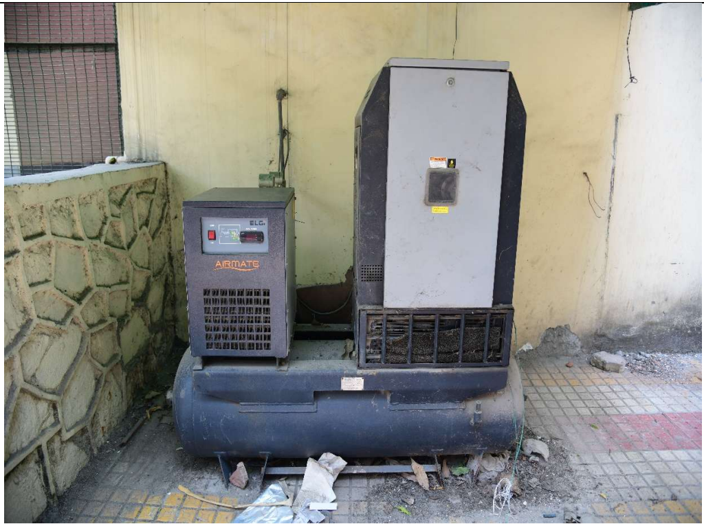
Elgi Air Compressor screw type with capacity 7.5 hp for CTP Machine
