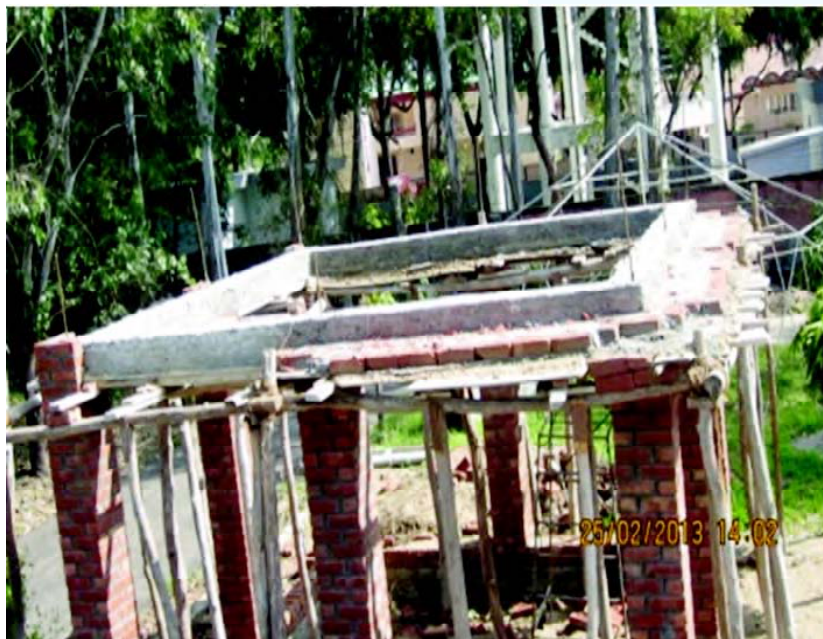
Fig. 1. Experimental models – Construction under progress
