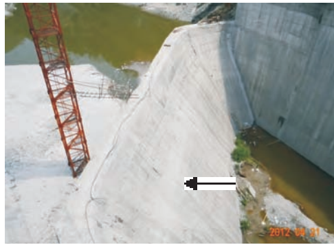
View of coffer wall from top of the Dam
