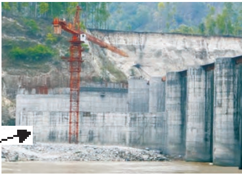
View of coffer wall from the upstream side of the river
