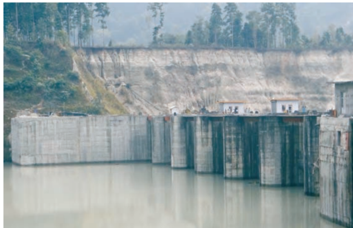
(a) Cellular wall and barrage pier
