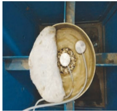
Fig. 2. View of stone column and location of earth pressure cells
