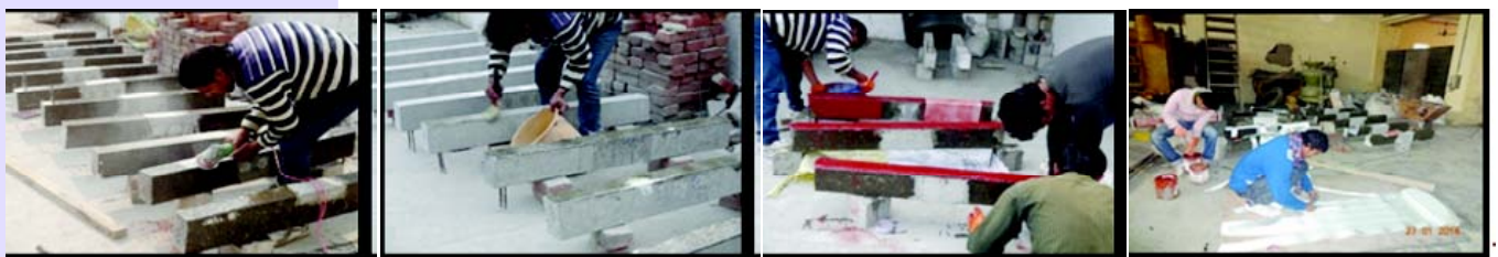
Fig. 3: Procedure for FRP application
