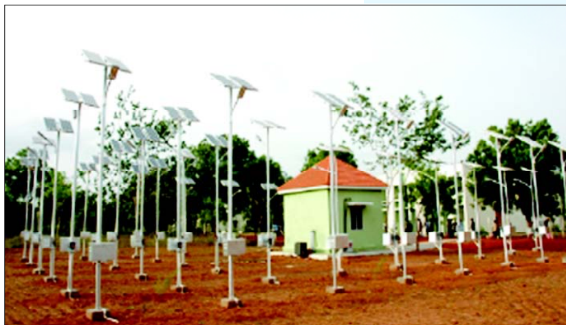
Photovoltaic Battery Testing Station
