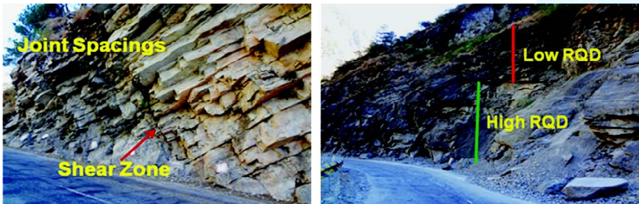
Fig. 2: Field observations of rock discontinuities
