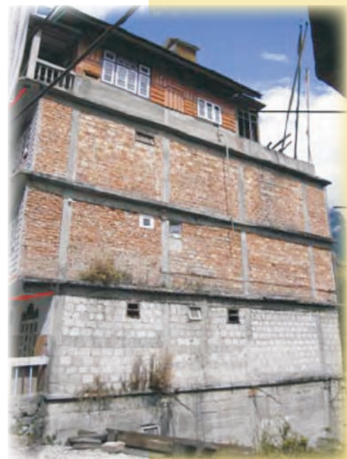
Figure 5: Typical hybrid infill RC construction in Lachung
