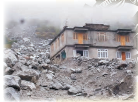
Figure 3: Damage due to mudslide at Lachung
