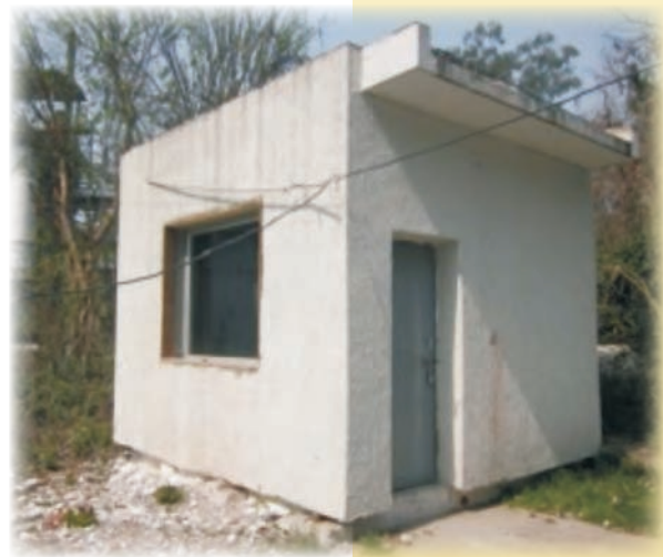
South facing treated window in room
