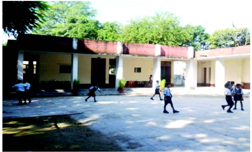
Photo 1: View of single-storeyed building adopted as a platform for demonstration of CSIR-CBRI technologies
