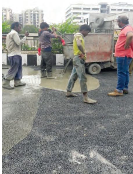
View of pouring of grout and squeezing on high voids bituminous mix
