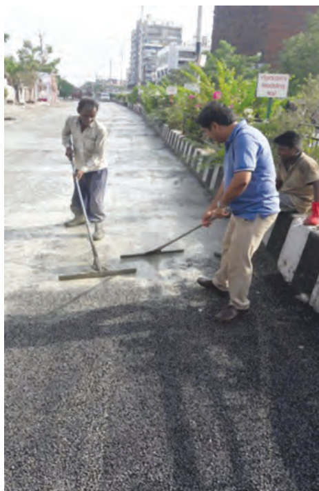
View of pouring of grout and squeezing on high voids bituminous mix
