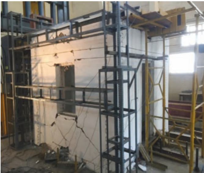
Fig. 2: Full-scale retrofitted confined masonry building subjected to lateral cyclic load
