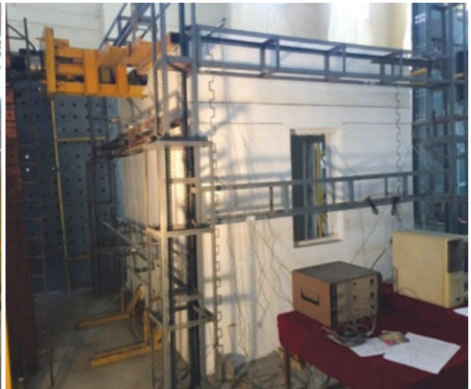
Fig. 3: Damage pattern for retrofitted confined masonry building subjected to lateral cyclic load
