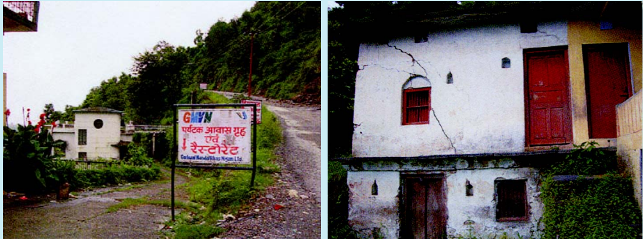
Fig. 2: Road subsidence and damaged houses
