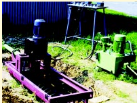
A view of underground horizontal boring machine
