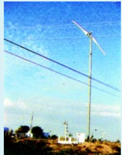
Fig. 8 — Wind turbine support tower
