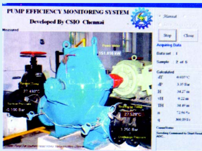
Pump Efficiency Monitoring System
